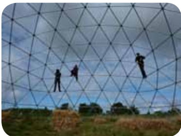
Team of international volunteers constructing the dome. Photo from Suderbyn Permaculture Ecovillage archives
