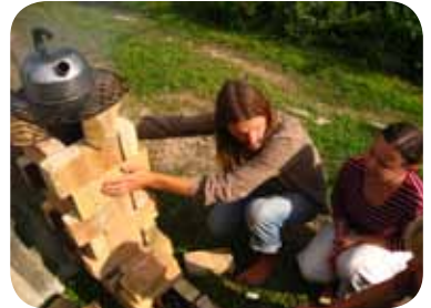
Learning by doing with garden kiln construction. Photo from parmainupilseta.wordpress.lv
