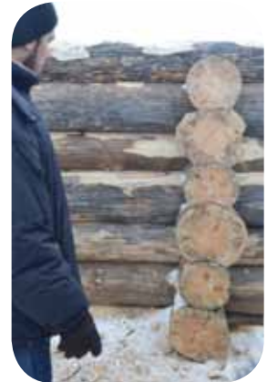
Working team from Kovcheg ecovillage construct houses using only axes according to traditional techniques. Photo by Irina Popova
