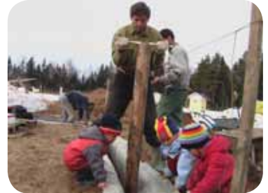
Building a house together. Photo from Kovcheg archives
